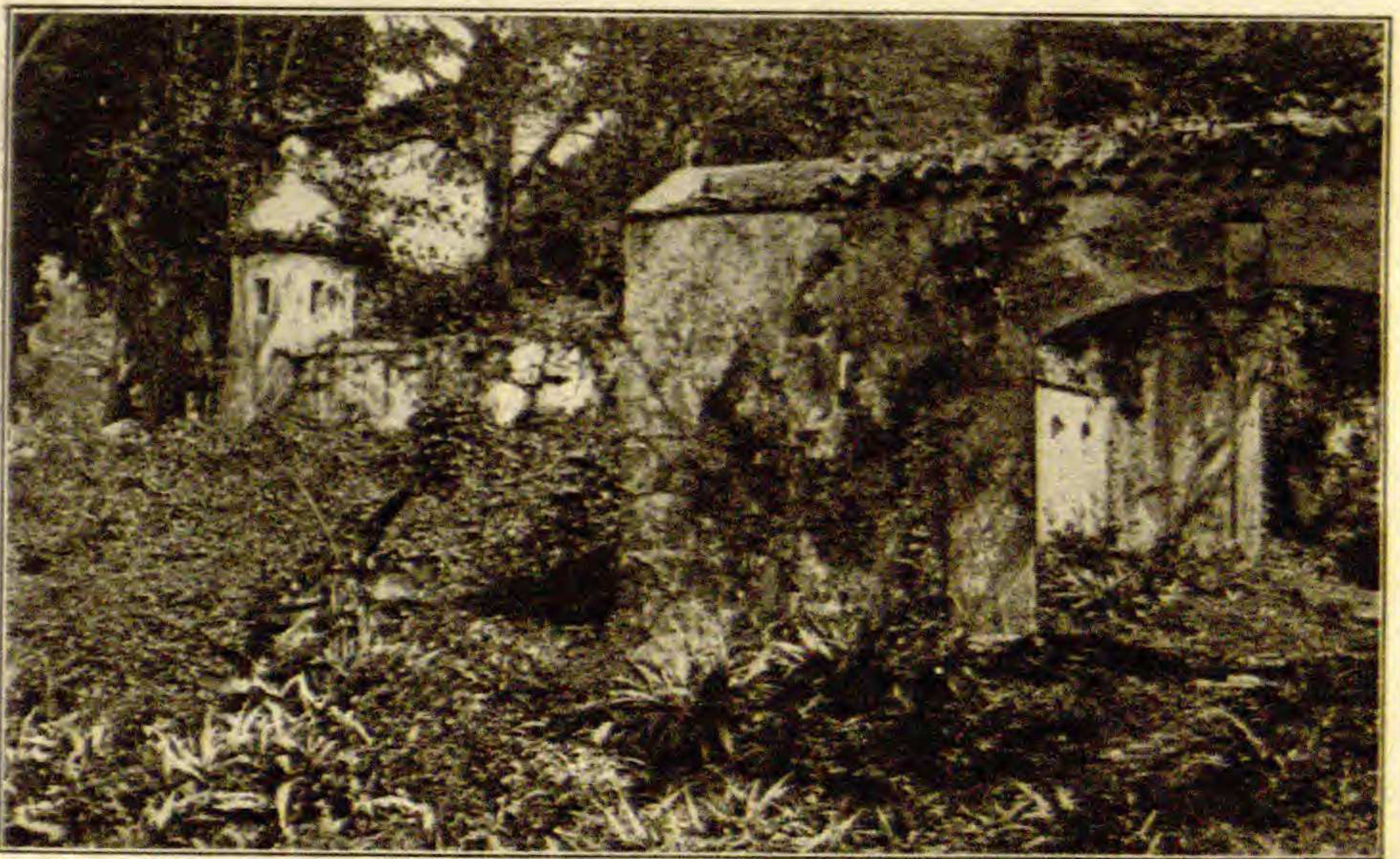
GATEWAY AND WATCH TOWER AT FORT SAN SEBASTIAN, PORTO BELLO, PANAMA
